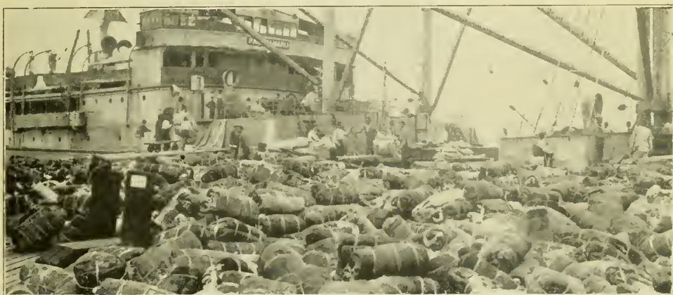
ABOVE: UNLOADING A LARGE SHIPMENT OF HIDES FROM SOUTH AMERICA
